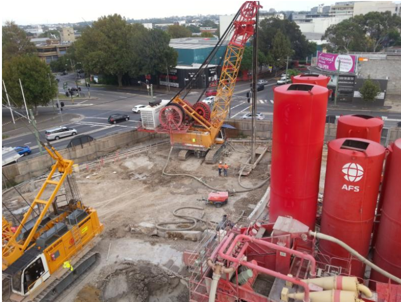
Construction of the diaphragm wall
