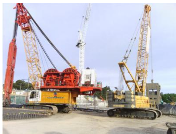
Hydrofraise used to build the diaphragm wall
