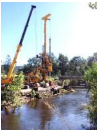
Environmental control at bridge site
