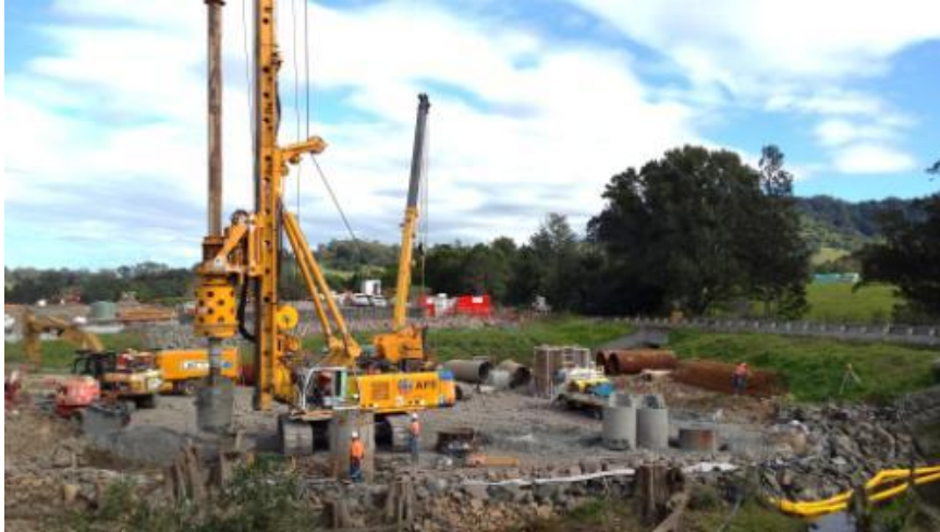
Broughton Pier piles
