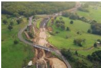
Tindalls Lane bridge site
