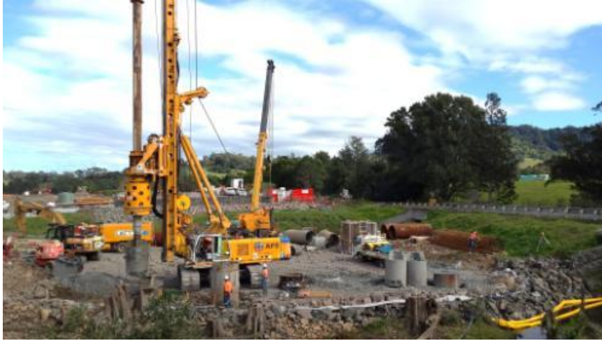
Broughton Pier piles
